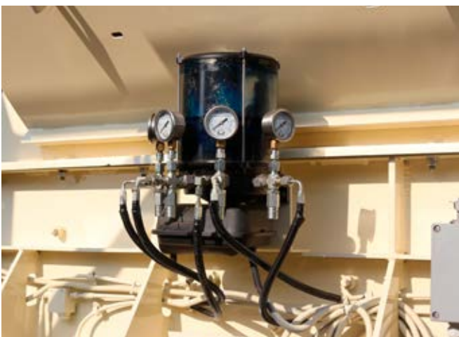
#5 Automatic Greasing System with pressure gauge on each delivery line
